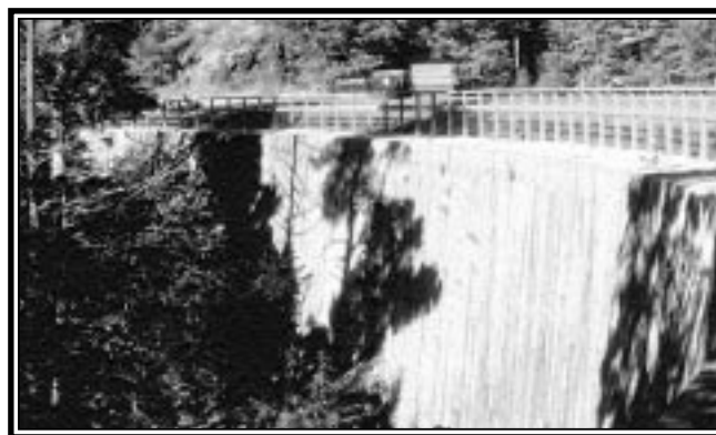
The Stone Arch Dam at Jones Falls, Rideau Canal Photo Collection.
