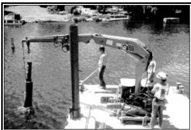
Setting navigation aids in the Canal near Manotick Rideau Canal Photo Collection
