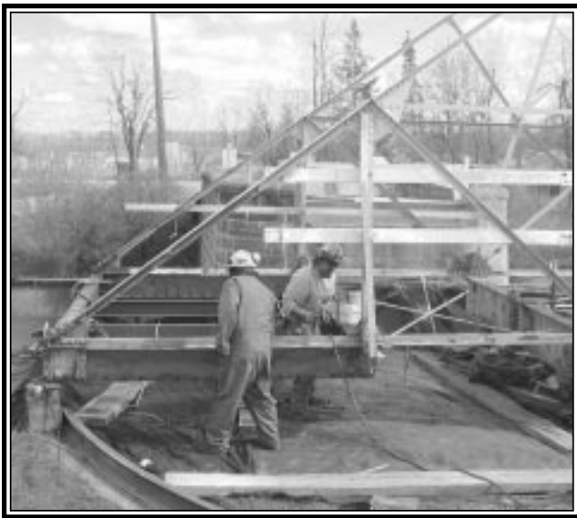
Burritt's Rapids Swing Bridge Bill Pratt
