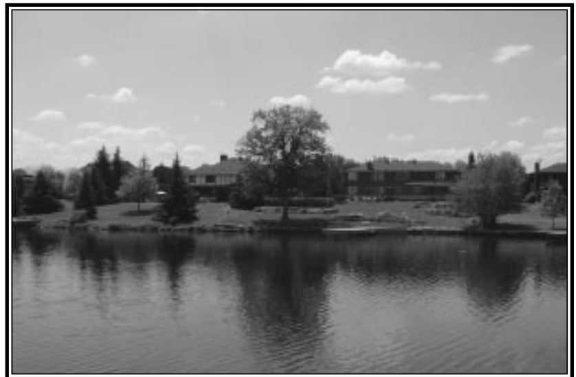
Suburban development is not consistent with the ecological health of the Canal environment.
